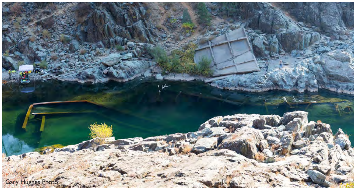
Photo demonstrates just some of the debris from the Highway 49 bridge that washed into the American River due to the failure of the Hell Hole Dam on December 23, 1964.
