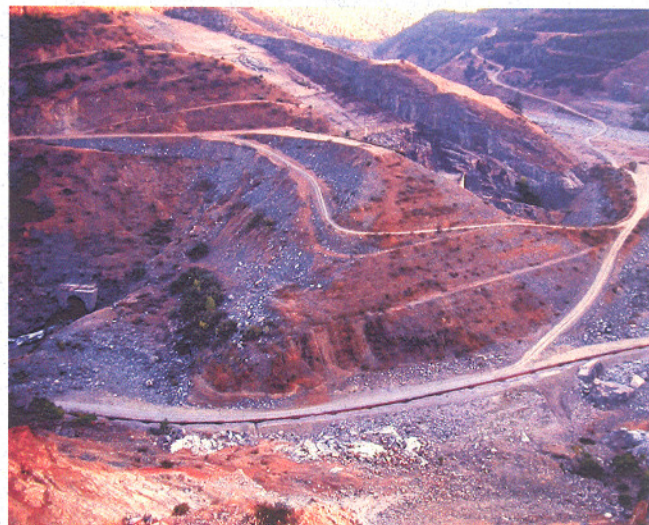
Auburn dam site 25 years after construction came to a halt due to seismic concerns. Photo by Mark Leder-Adams
